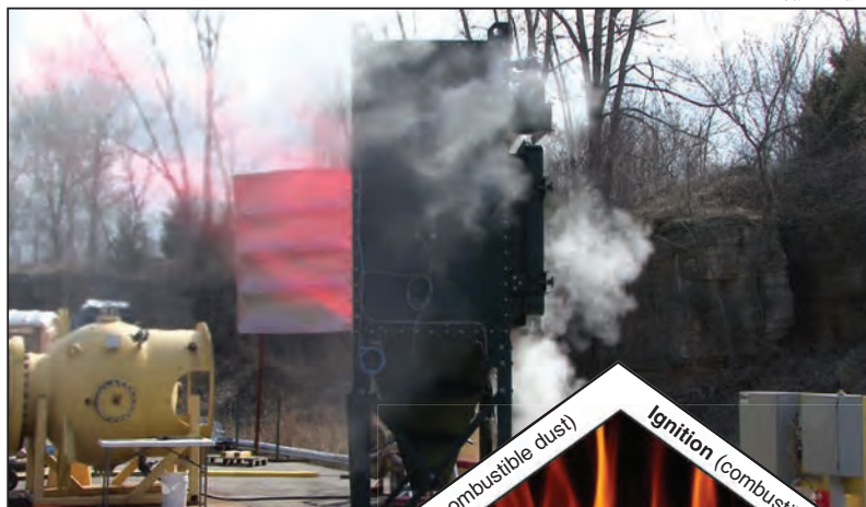
FIGURE 1. This image was pulled from a video of an actual staged explosion that was performed to test whether a dust-collector explosion vent would work as intended. It did. The explosion vent, which has popped open here, is designed to relieve internal combustion pressure to keep the collector from blowing up into pieces. The collector will typically experience internal damage in an explosion like this, but if personnel remain safe, the explosion protection system has done its job
